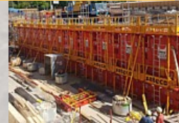
Chantier rond-point SERRA
